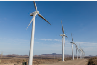
TURKANA WIND FARM
