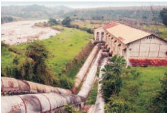
SANGA POWER PLANT
