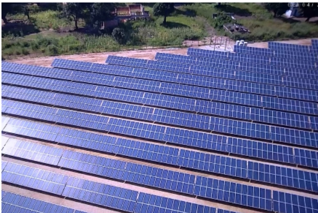
AERIAL VIEW OF THE POWER PLANT
